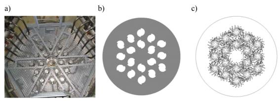
Fig.3. Set of EV burners in silo-combustion chamber (Badur et al., 2004):
