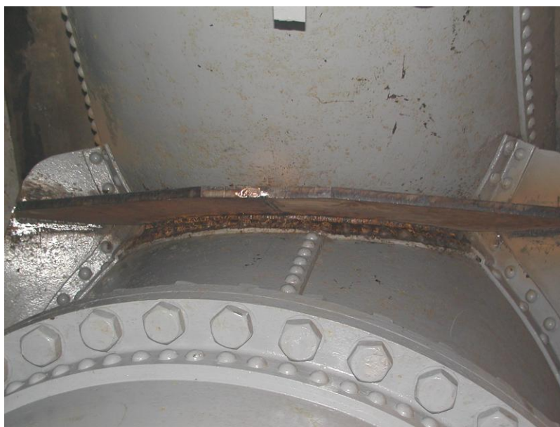
Fig. 3 Strengthening fin at pipeline branching
