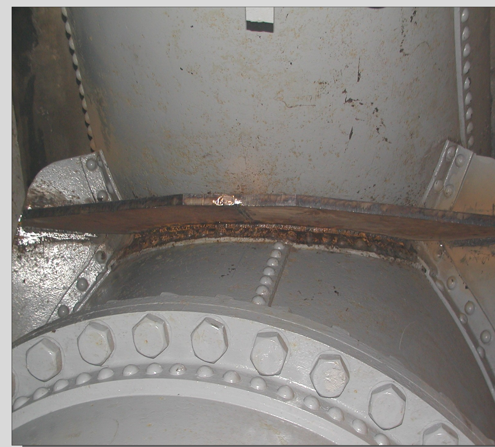
Fig. 3. Strengthening fin at pipeline branching.
