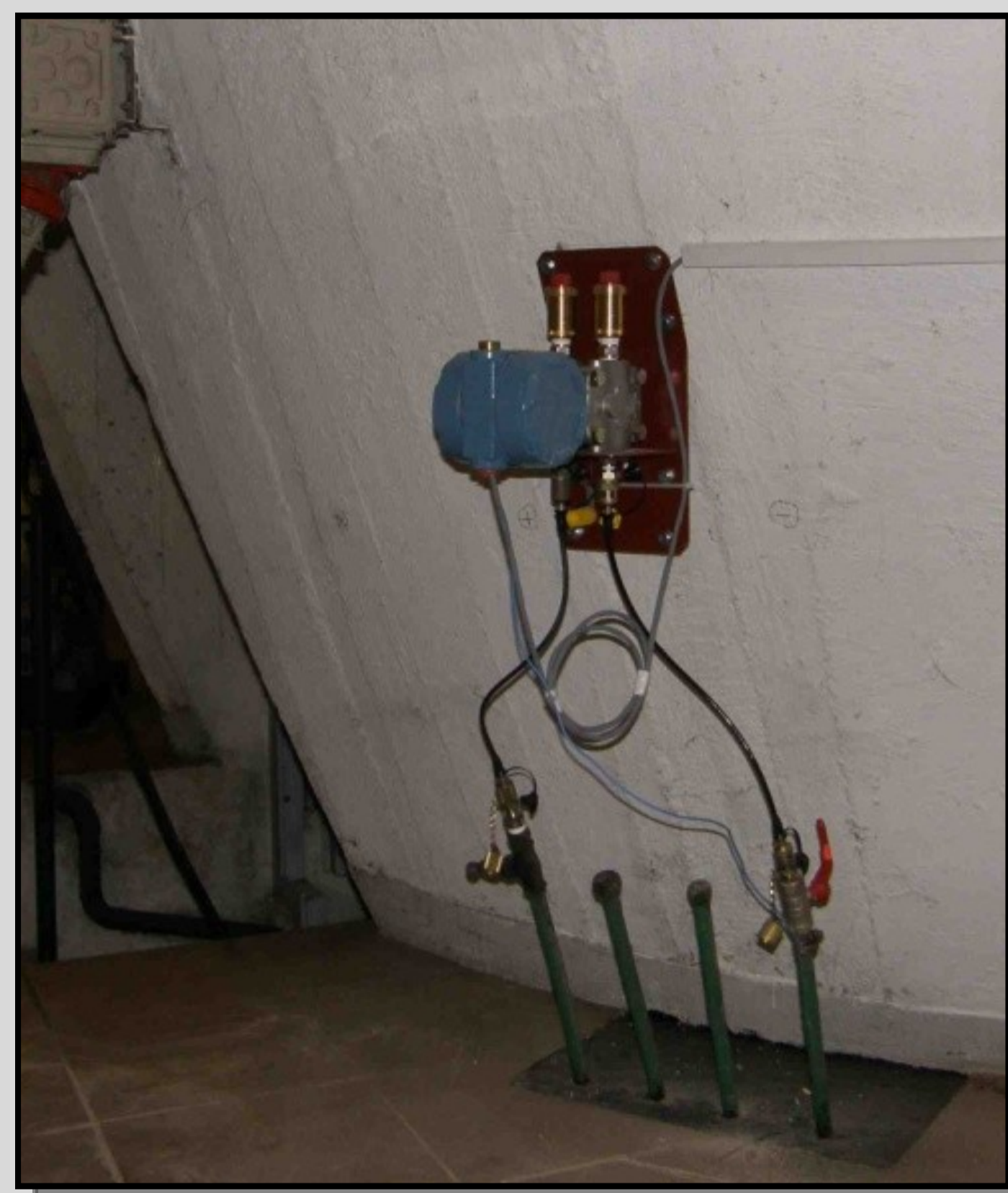
Fig. 2. Differential pressure transducer for continuous flow rate measurement equipped with the automatic venting system.
