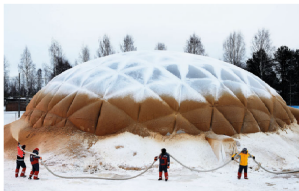
Figure 14: Making of a pykrete dome [9].
