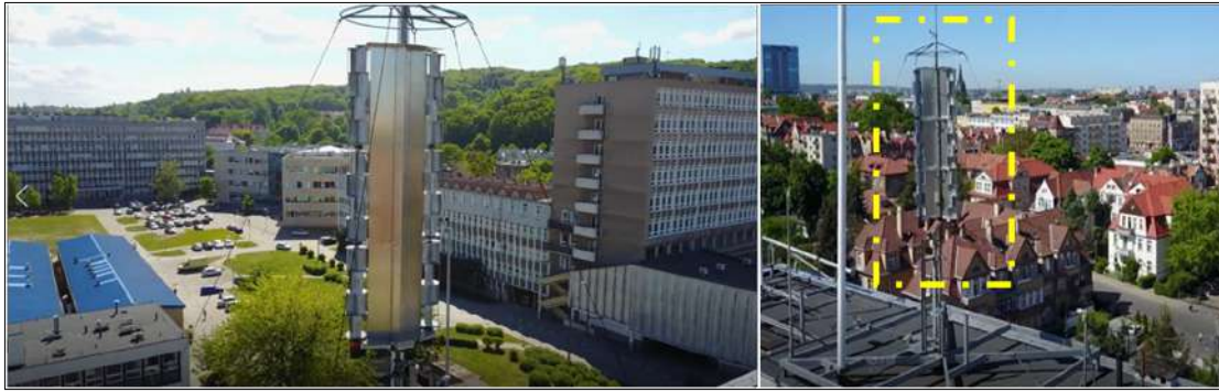
Figure 5.2.1: Innovative WT prototype on the roof of IMP PAN building
