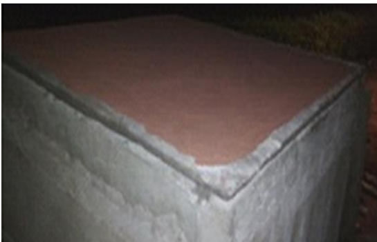
Fig. 5. Rubber sheet roof slab.
