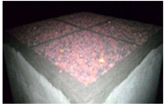
Fig. 7. Roof slab with Jhama brick bats.
