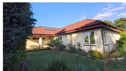
Fig. 2. View of the analysed building.
